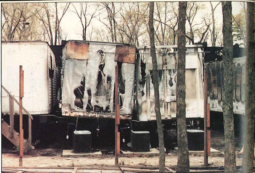
From left to right, the rear of the spider, frankenstein, and strobe room trailers (the latter being the point of fire origin) show the effects of the heat generated. The air circulating units that intensified the fast-moving fire are located in the foreground.
